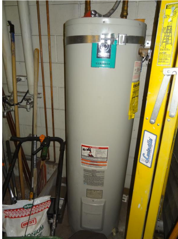
Washoe Casual Labor Office - Building #1473 Description: Water heater replacement needed.
