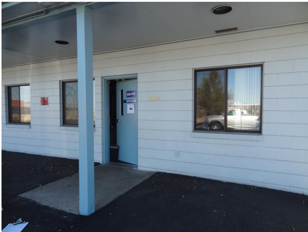
Washoe Casual Labor Office - Building #1473 Description: Window replacement needed.
