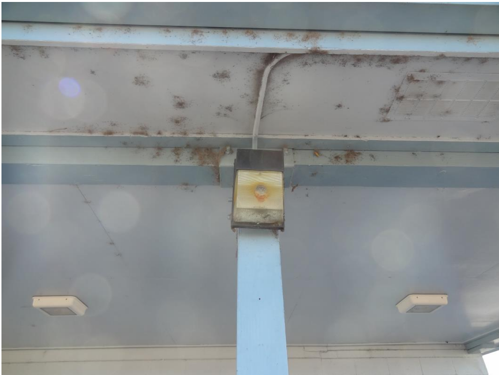
Washoe Casual Labor Office - Building #1473 Description: Exterior lighting replacement needed.
