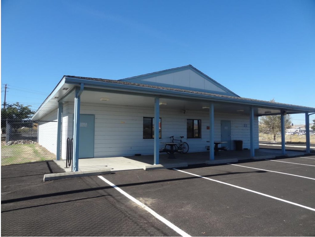
Washoe Casual Labor Office - Building #1473 Description: Exterior finishes.
