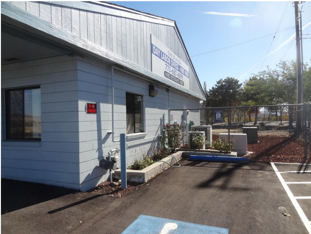
Washoe Casual Labor Office – Building #1473 Description: Seismic gas shut-off valve installation needed.
