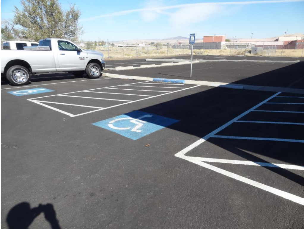
Washoe Casual Labor Office – Site #9847 Description: ADA accessible path of travel needed.
